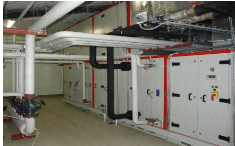
We perform connection and installation of equipment
