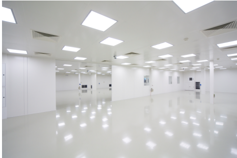
Supply and installation of clean room structures
